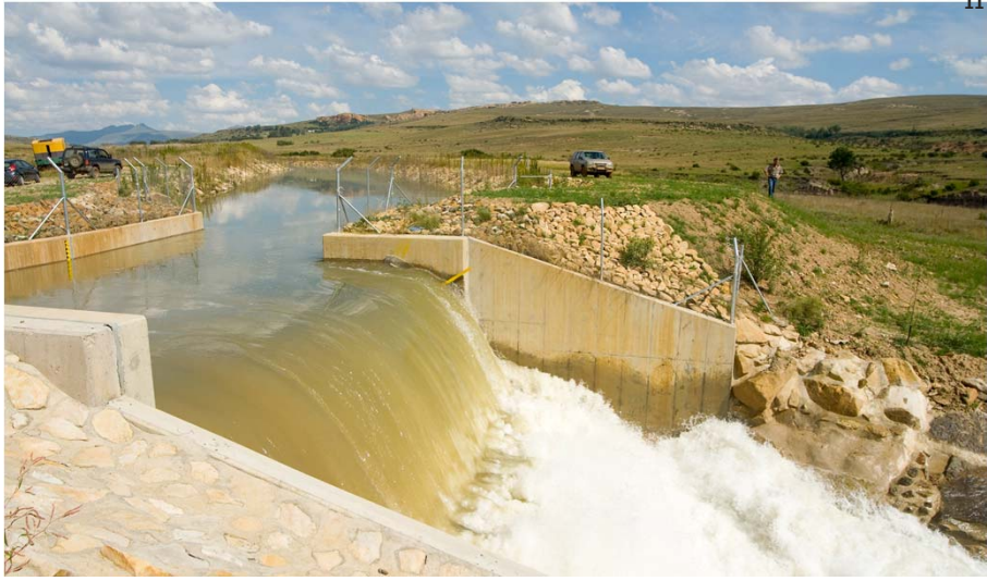
Spillway in use
